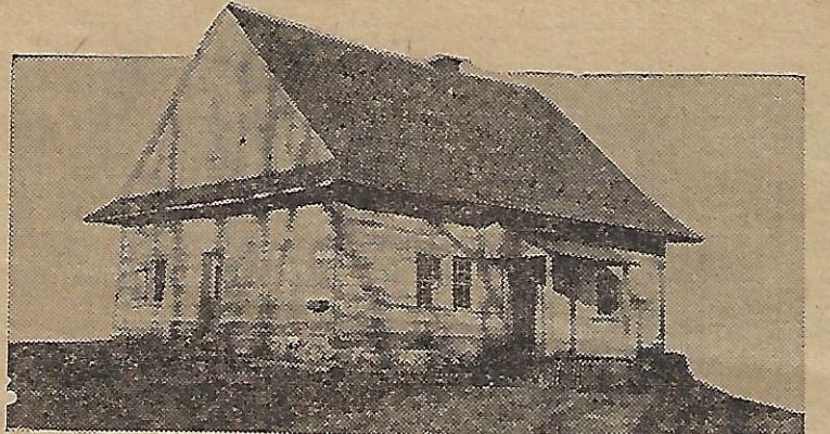
The old Mennonite Meeting House at Landisville, which is said to have been built in 1740.
